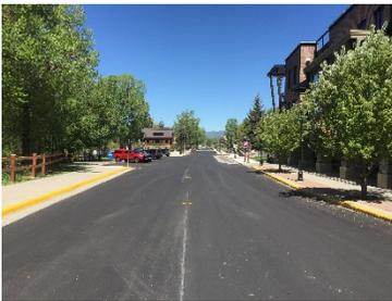
Paving on Yampa Street was completed earlier this week. The entire stretch of the road was milled and paved from 5<sup>th</sup> to 12<sup>th</sup> Streets. The paving portion completes the final major enhancement to Yampa Street during the three year improvement project.
