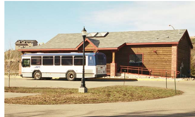
Stockbridge multi-modal center
