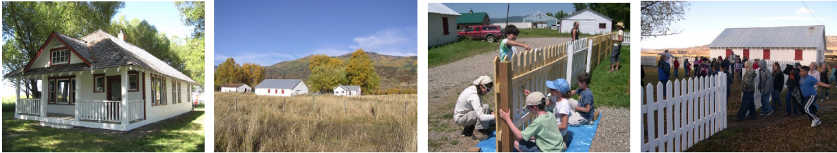
Main House, c. 1917; Bunk house, not shown, c. 1929; Coal Shed, c. 1920s; Barn, c. 1960; Pole/Stock Shed, c. 1945
