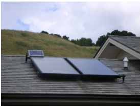
M.7 Install Solar Water Heating System
