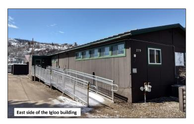
The building has wood siding and a pro-panel metal roof, set on cinder block piers and is supplied with public utilities such as natural gas, electricity, and municipal city and sewer service. Set on a foundation, the mechanical building is a wooden structure measuring 26' x 26' with a metal single shed roof rising measuring 10'H to 18'H.
