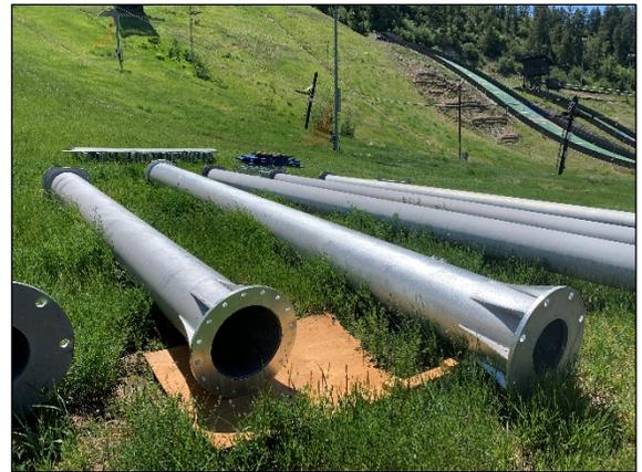
Joining SkyTrac on the hill is GeoStabilization International, a slope stabilization contractor. Crews have been installing soil anchors above lift towers 3, 4, 6 & 7 on the hill. In addition, micro-piles up to 40-foot deep are underway. These will be connected directly to the lift towers foundations to increase stabilization.
