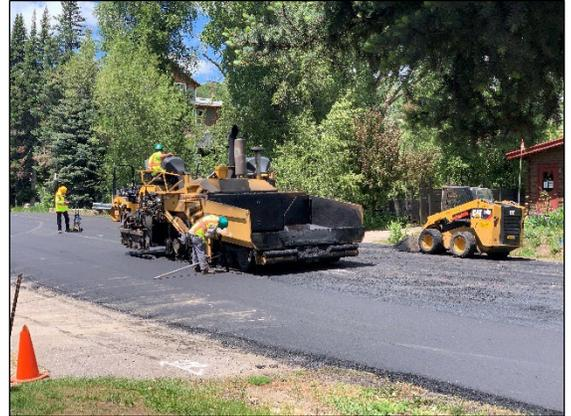
In addition, the project covers just over 450,000 sq ft with a two-inch lift, typical across the region for strength requirements associated with traffic loading. Weather permitting, paving should take five days to mill and two weeks to fill with new asphalt.
